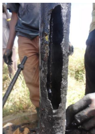
(c) Removal of corroded pipes Source: Richard Carter.
