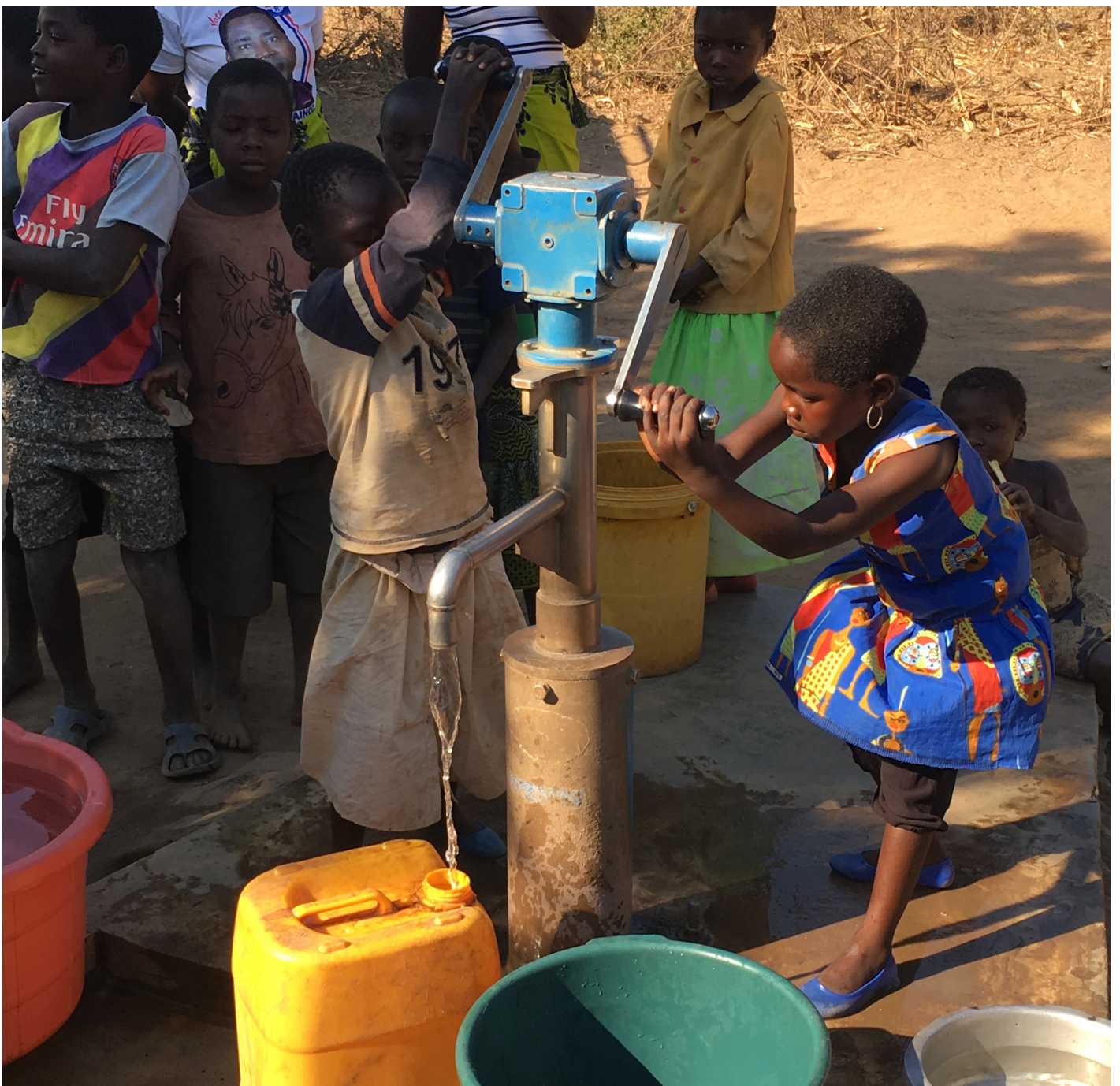
Figure 10: Second LifePump installed in Chilekwa Village, Kasungu District, Malawi, August 2018
