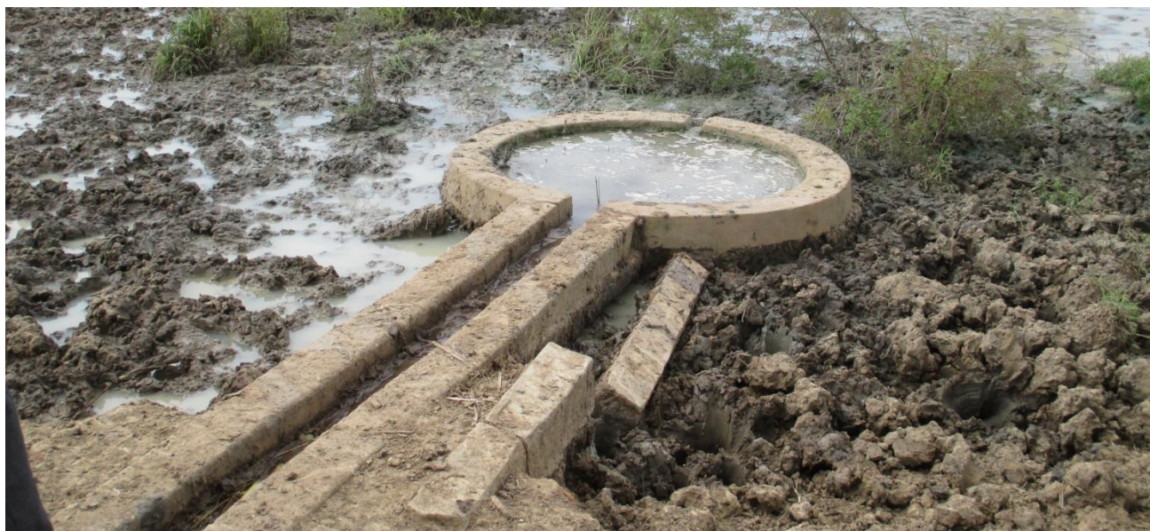
Figure 6 Drainage channel and cattle trough from handpump close to Aweil Town after several rehabilitations
